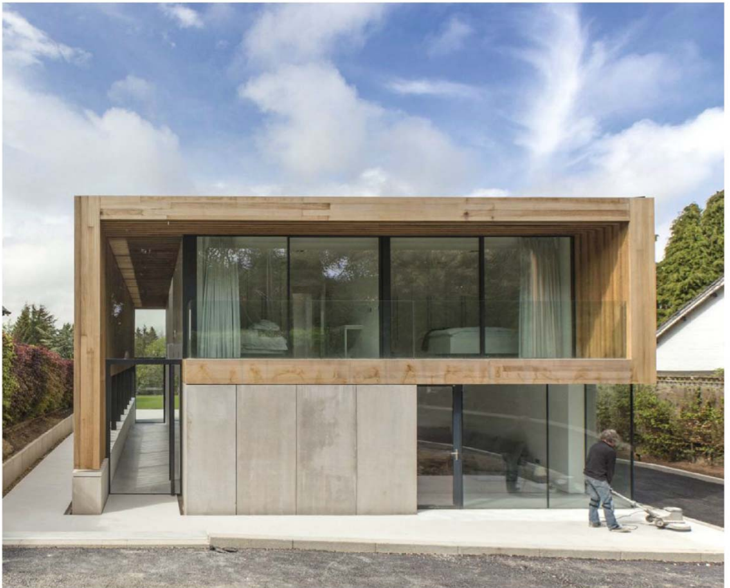
▽ Front elevation. Shielded from solar gain by an external FSC-certified hardwood timber screen, full-height windows and rooflights provide good levels of daylight throughout the plan.
