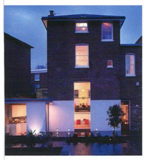
Grade II listed house in north London that he extended into a rear garden over two floors, opening up the views and bringing light deep into the property. "We built a big, structural glass box in which the glass walls carried the weight of the glass roof, which itself was one huge panel of a new type of glass [Pilkington's Suncool] that won't overheat in summer," he says. And even where
