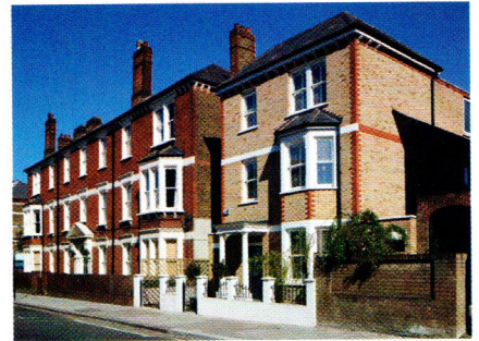
John Osborn Design Bricks laid in Flemish bond and sash windows complement the neighbouring Victorian homes
