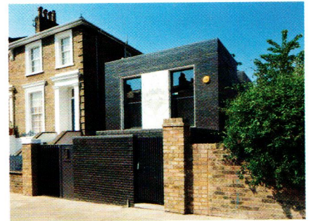
Liddicoat & Goldhill Born out of the constraints of a small site, this striking home uses a flat roof to minimise its impact
